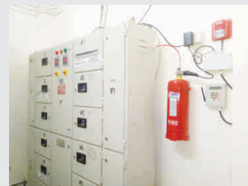
FIREDTK Tubing Installation
